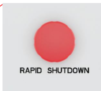
Figure 5.19 Rapid Shutdown & Emergency Power Off Initiation Switch
