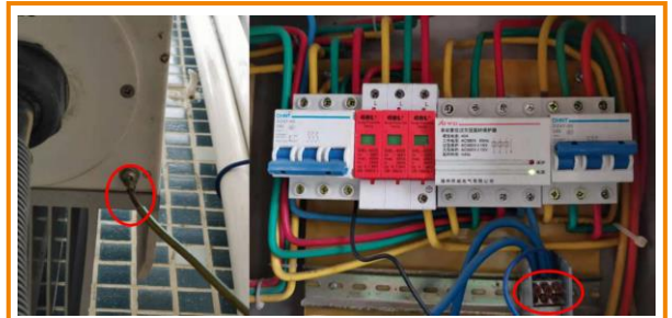
Figure 2: Corroded PE cable and grid box interior
