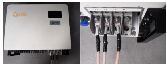
Figure5: Cu-Al Wire Connector
