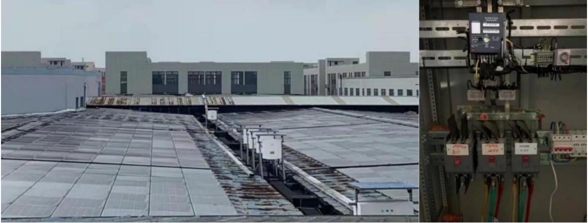
Figure 3: On-site PV+ diesel generator set hybrid power supply scheme
